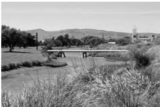
Figure 10.14 – Sewerage crossing Waikanae Creek
