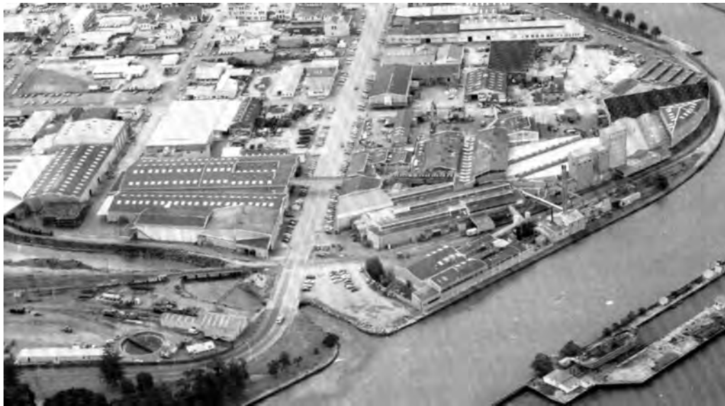
Figure 10.7 – The Watties site, straddling Customhouse Street 199 .
