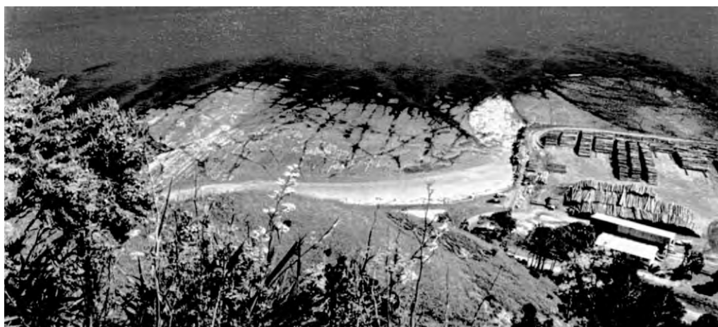
Figure 6.9 – Encroachment of reclamations onto wave platforms
