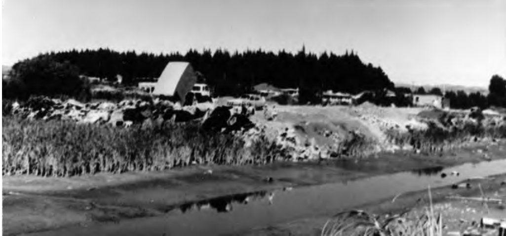
Figure 8.13 – ‘Controlled tip’ encroachment on raupo Stanley Rd., late 1961 261
