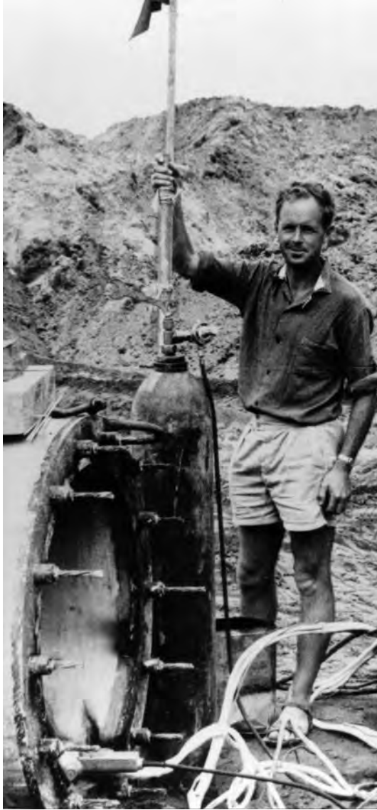
Figure 11.1 – H.C. Williams, Chief Engineer, GCC, 1957-1986, pictured during construction of the submarine sewerage outfall.
