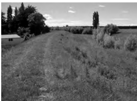
Figure 4.6 – A stopbank on the Whakaahu Stream
