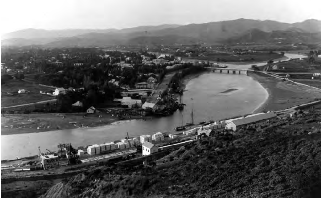
Figure 6.3 – Reclamation of mudflats: 1891 vs 1909 a
