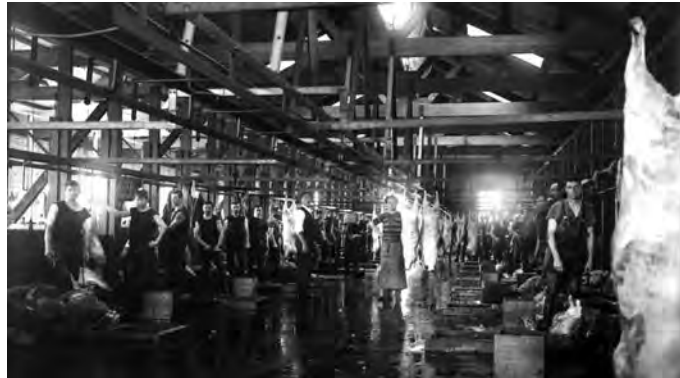
Figure 10.4 – Insanitary conditions inside the Kaiti works, 1913 120 .
