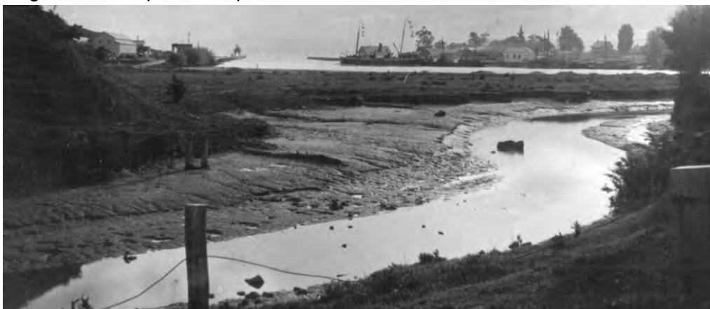
Figure 6.6 – Kopuawhakatapa Creek 1905, before the culvert and reclamation 130
