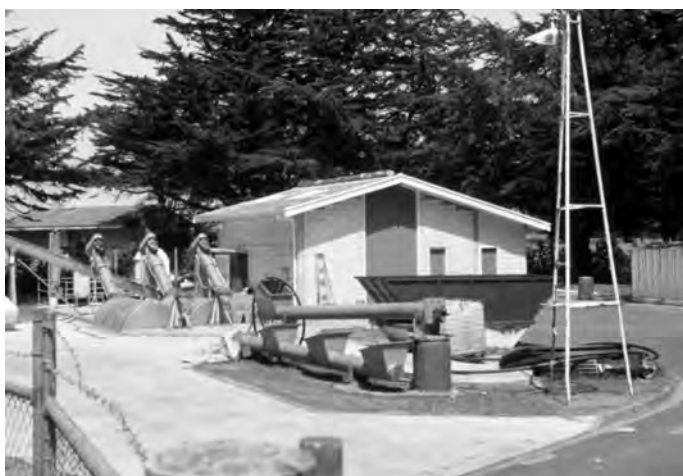
Figure 11.2 – Gisborne sewage pumping station with milliscreens at left.
