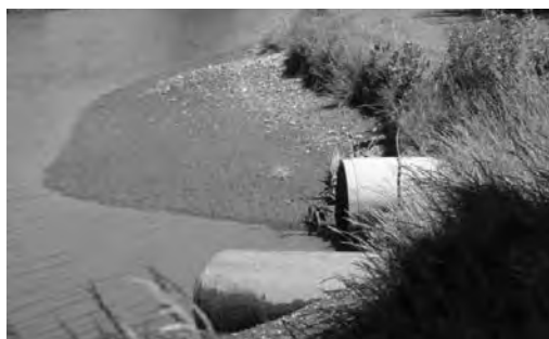
Pipes flowing into Waikanae Creek – these flowed through old landfills and carried unspecified 'stormwater' into the Creek.
