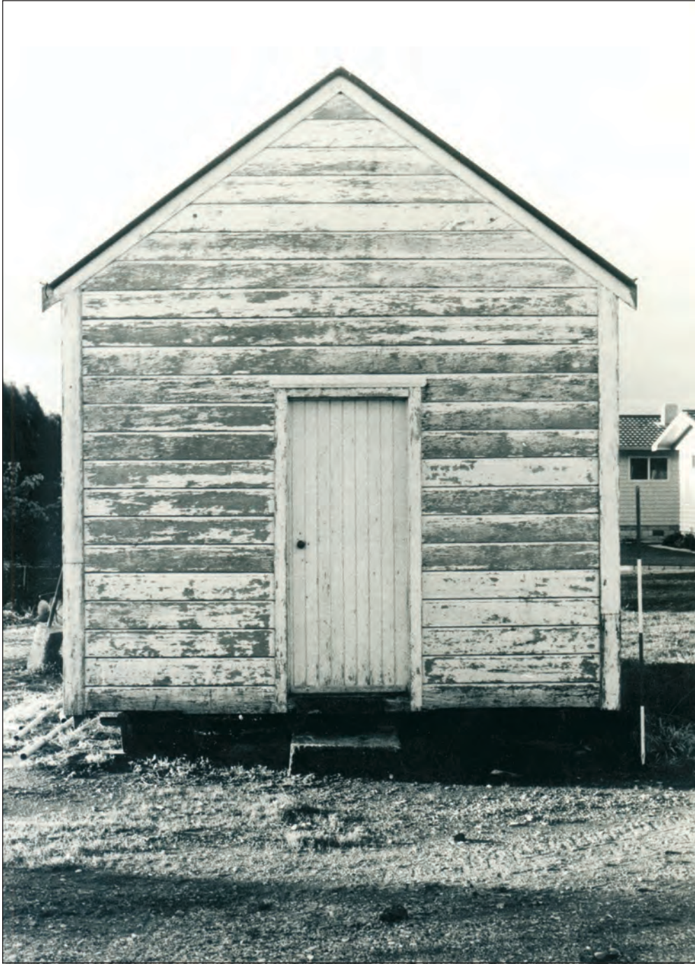
Fig 14: Sled house. Photographer unknown. Reproduced courtesy of the Tairāwhiti Museum, Gisborne, New Zealand (1978-601-14). The notice beside the sled house, which stands outside the Tairāwhiti museum, reads: 'The runners underneath allowed the house to be moved by a team of bullocks. This was needed in the 1870s when land possession was uncertain, floods frequent and fear of Hauhau uprisings general. The house's last site was in Bushmere Road.'
